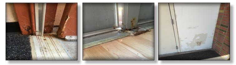
▲ Several sets of exterior doors have deteriorated due to age and exposure to salt that is used for de-icing. Doors that are in poor condition are difficult to close at times and could pose a security risk.
