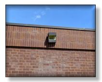
◄ The exterior lighting is obsolete and low efficiency. The payback on utility costs and maintenance savings of new LED lighting is very favorable. The exterior lighting should be upgraded before any major repairs or maintenance is performed on the existing fixtures. ►
