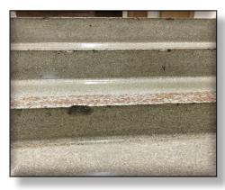
The concrete steps and sidewalks surrounding the building need to have cracks repaired, uneven pavement leveled, and curbs should be painted yellow to let people know that there is a step according to applicable codes to avoid trip hazards. ►
