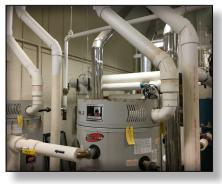
◄ The existing domestic water heaters need to be repaired or replaced. Based on the reliability of the existing water heaters, the more cost efficient option is most likely replacement.
