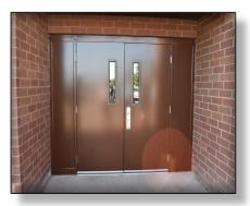
✓ Even though these are commercial doors and have been well maintained, when they have been used for 30 years, they will have issues. The doors that are original should be scheduled for replacement.
