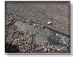
◄ The roof can be replaced with the same type of rubber roof with the rocks over the top (ballast), or it can be converted to a fully adhered roof. The ballasted roof is the more economical option, but the rocks on top of the roofing material make it difficult to find leaks when they happen.
