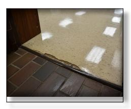
✓ Wherever there is a transition for the flooring, such as the transition from a doorway to a classroom or from carpeting to vinyl tile in the middle of the classroom, there are issues with the flooring being in poor condition. The vinyl tile throughout the building has been damaged or is peeling because of years of use. The carpet in the classrooms has also surpassed its predicted useful life and needs replacement to address areas that have trip hazards or are excessively worn. ►
