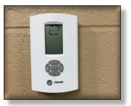
◀ The thermostat for the office air conditioning has a malfunctioning display and cannot be programmed. The thermostat needs to be replaced.
