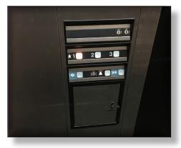
✓ Due to its age, there aren't any replacement parts available for the elevator. This is a major concern, because if the controls malfunction, the elevator will be out of service for an extended amount of time. ►
