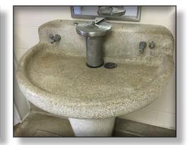
▲ The hand wash stations and the oldest sinks need to be replaced. They are difficult to adjust and parts are becoming obsolete.
